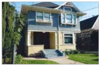
WESTON HOUSE 2112 Portland Street
